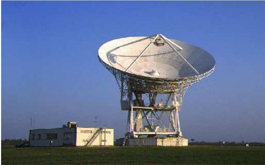
**Fig. 1.** The 32-meter diameter telescope of the Istituto Nazionale di Astrofisica (INAF). It is located near Medicina, close to the Adriatic Sea. Picture taken from the 2009 International VLBI Service for Geodesy and Astrometry (IVS) Annual Report by Orfei et al. (<http://ivs.nict.go.jp/mirror/publications/ar2009/nsmedi/>)
