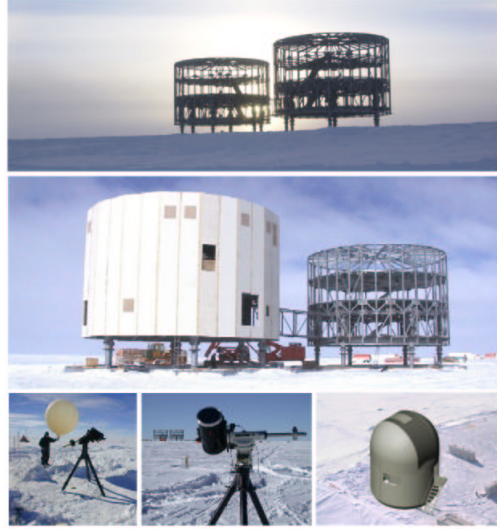
Fig. 4. The two main buildings of the Dome C base under construction, preliminary site testing and a pictorial view of the IRAIT dome.
