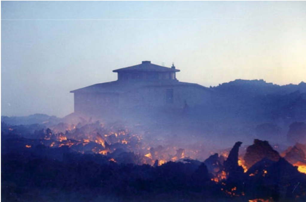
Fig. 3. Vincenzo Bellini Observatory surrounded by the 1971 lava flows, few days before its complete coerture. It is possible to note the skylight built to replace the dome when the astrophysical observatory became a volcanological one.
