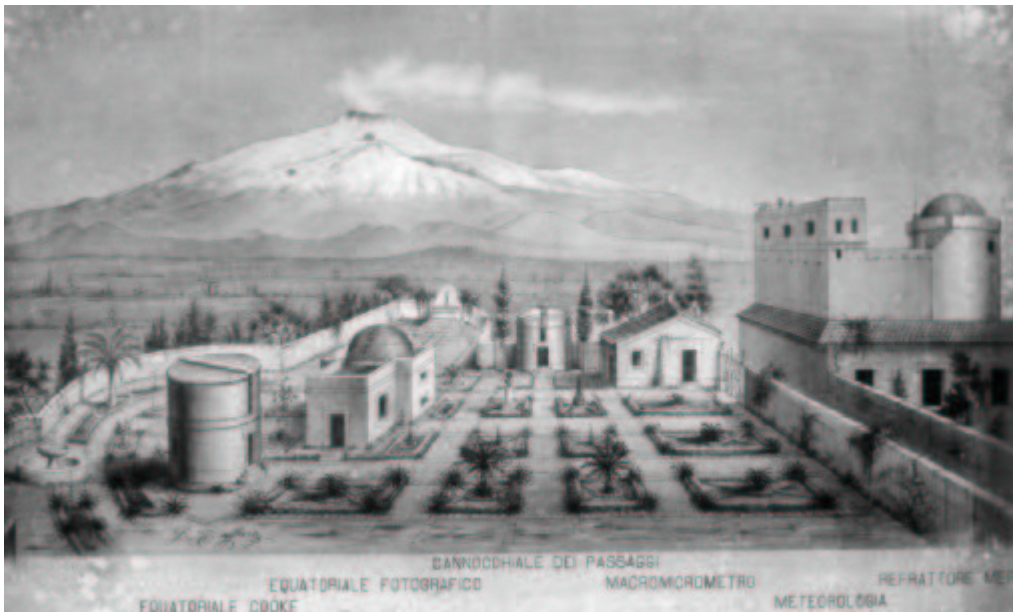
Fig. 7. An old stamp of Luigi Taffara's that represents the pavillions built in the garden near the Benedettini Monastery. On the left the dome of the 15-cm aperture and 2230-mm focal length Cooke equatorial refractor, the 33-cm aperture and 3341-mm focal length astrograph (manufactured by Steinheil of Bayern Munich and with an equatorial mounting realized by Salmoiraghi factory of Milano) and the 9-cm aperture meridian circle; on the right the tower of the Merz dome. The Carte du Ciel , the first photographic Catalogue and Atlas of the entire heaven vault, promoted by the France Academy was realized using the Steinheil astrograph.
