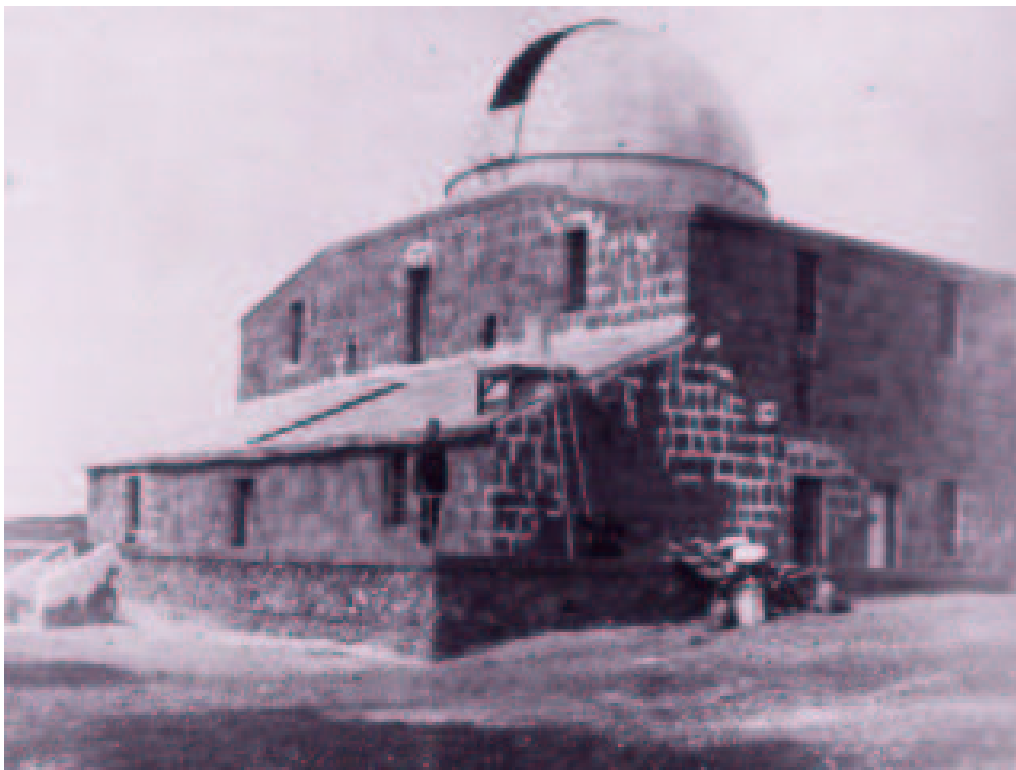
Fig. 1. The Vincenzo Bellini Observatory built near the Etna central crater at 2941-m a.s.l.. The main telescope of the new Observatory was a Merz refractor having a 34-cm aperture objective, 5570-mm focal length and an equatorial mounting by Cavignato of Padova, with iron pipe. The dome was ordered from Oretrea factory of Palermo.
