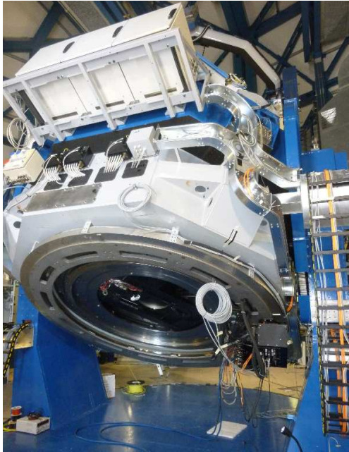
Fig. 4. The primary mirror cell integrated in the telescope (September, 2010). In the bottom part the guide probe is visible, as well as the technical CCDs controllers and the co-rotator control cabinet.
