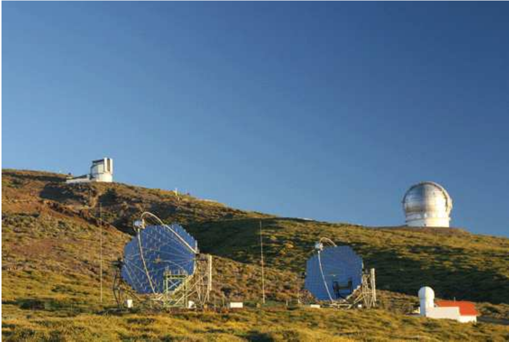
Fig. 2. A picture of the MAGIC array consisting of two 17 m diameter Cherenkov telescopes, in the foreground, the TNG and GranTeCan telescopes in the background on the left and on the right, respectively. They are located at Roque de los Muchachos, 2200 m a.s.l., La Palma, Canary Island.
