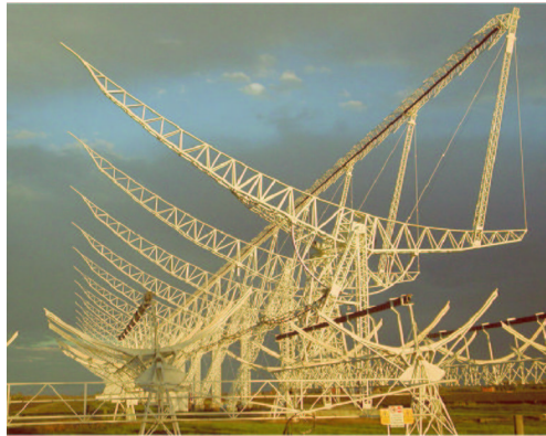
Fig. 3. The large Northern Cross Array, 560 meters (East-West arm) x 640 meters (North-South arm).
