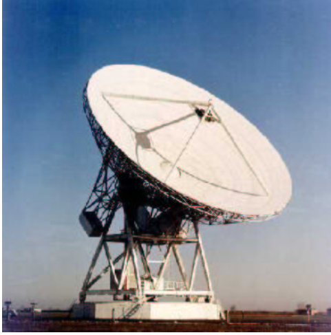
Fig. 1. Noto radiotelescope, a 32-m reflector antenna with active surface.
